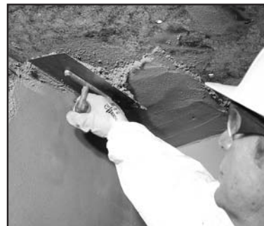
Working overhead is easily done
